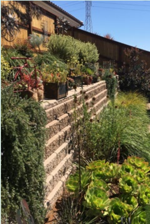
Retaining wall in the Kleinmans' garden
